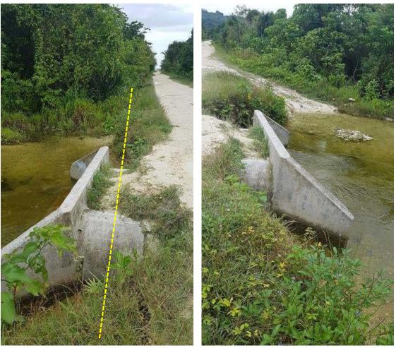
Figure 4-12 Cable crossing at Langa Langa freshwater lagoon
