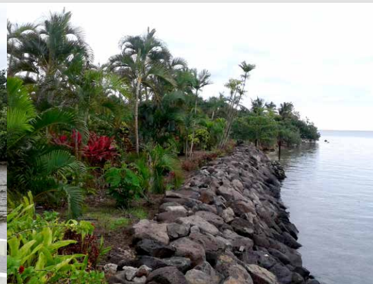
Removal of mangroves impacts on fish stocks and coastal stability, installation of stone seawalls for coastal protection needs to be carefully planned and assessed through a robust EIA prior to implementation, to ensure they will effectively protect community assets and not cause unintended impacts along neighbouring areas of coastline. Photo: Greg Barbara
