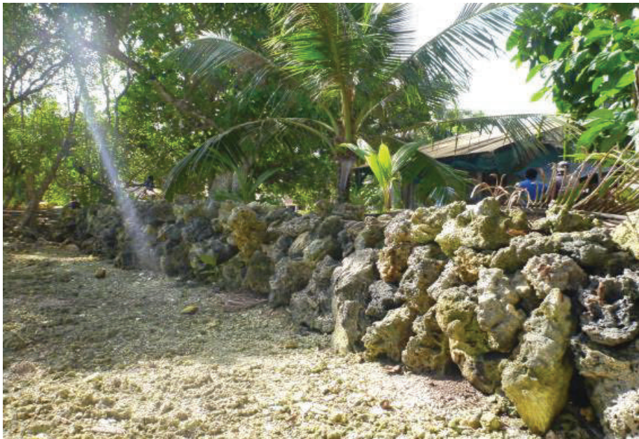
Figure 5-23 Coral rock used to construct a seawall
