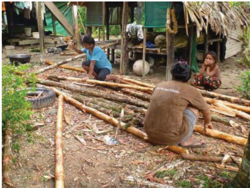
Figure 5-14 Preparation of mangrove timber for house construction or maintenance
