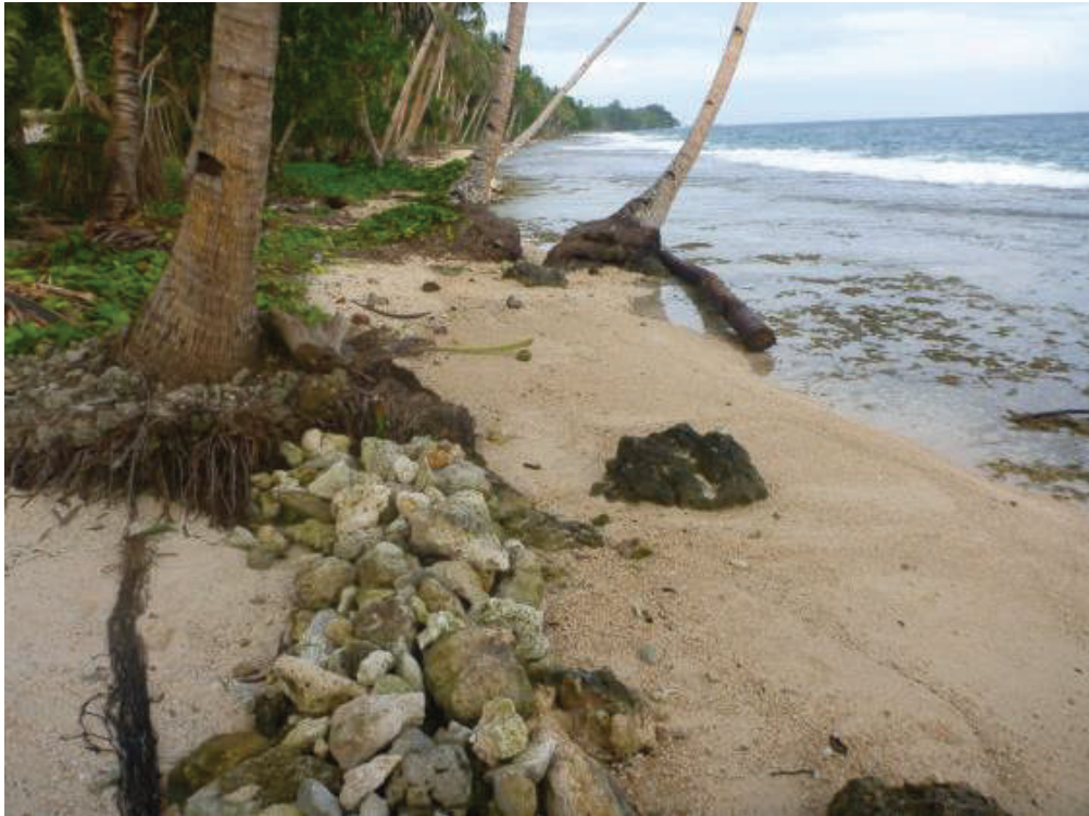
Figure 5-38 Coastal erosion and a small seawall along the sandy foreshore at Nikumaroro Village
