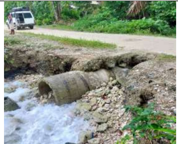
Plate 15 (Top and Bottom): Culvert and Roads being inundated by the sea in Ward 7, North Malaita. Courtesy by WECS, Sept 2021
