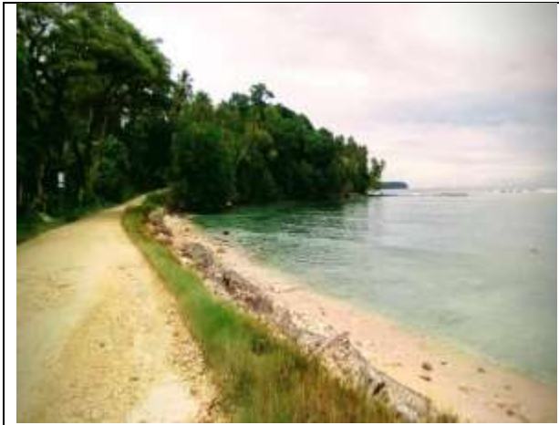
Plate 14 (Top and Bottom): Gabion being eroded by high waves, Ward 8, North Malaita. (Photo by WECS,2021)
