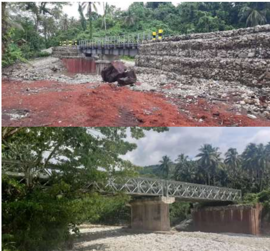
Figure 4: Newly repaired Taba'a (bottom) and Kwai (top) Bridges
