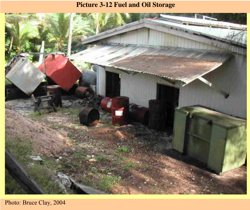
Picture 3-12 Fuel and Oil Storage
