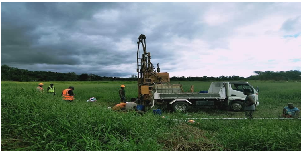
Fig 8: Drilling works on site for the Geotech assessment.
