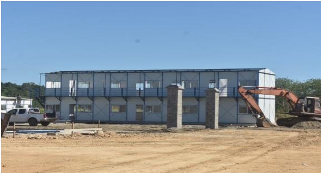
Fig 11: Temporary office sites for the construction, Mamara.
